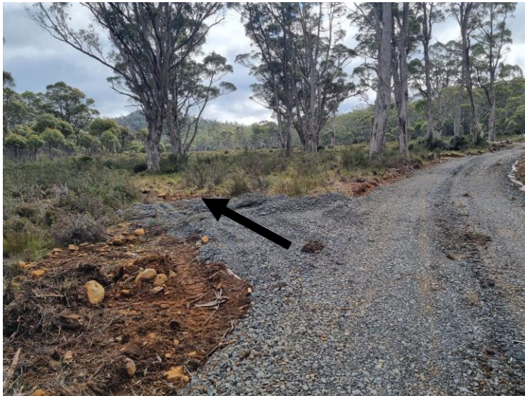
Image 5.1.2 – Access to units from main access carriageway
