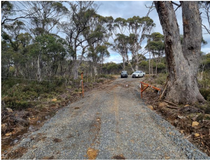
Image 5.1.1 - Main access under construction towards Lyell Highway
