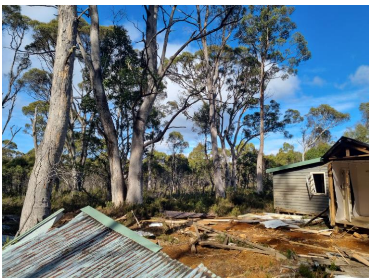
Image 4.1.7 – View SW across building area.
