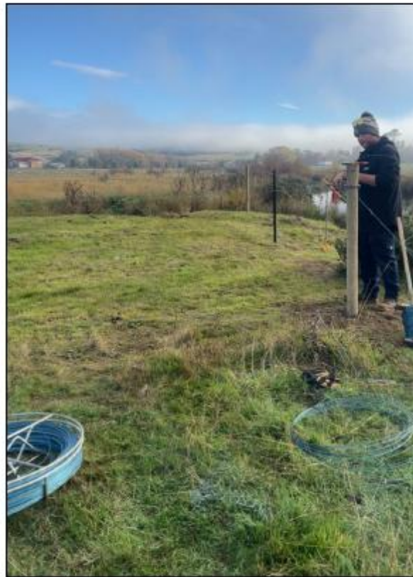
Figure 8. Ouse River restoration project fencing installation
