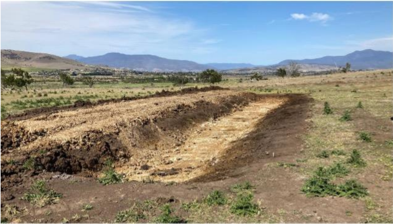
Figure 7-1: Biosolid stockpiling bund. Trucks unload on the right-hand side and the excavator loads the spreader on the left. A small berm on the loading site is added (not shown in picture) to prevent surface water entering and to provide a stop for the back wheels of the trucks (photo provided by Spectran).
