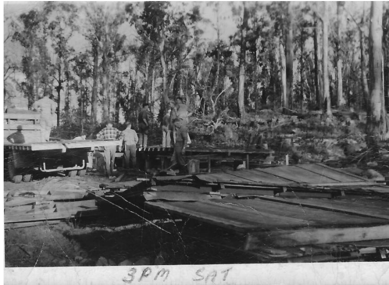
Floor section of shack re-laid on stumps, Dee Lagoon, Saturday 4 October 1958, 3.00 pm
