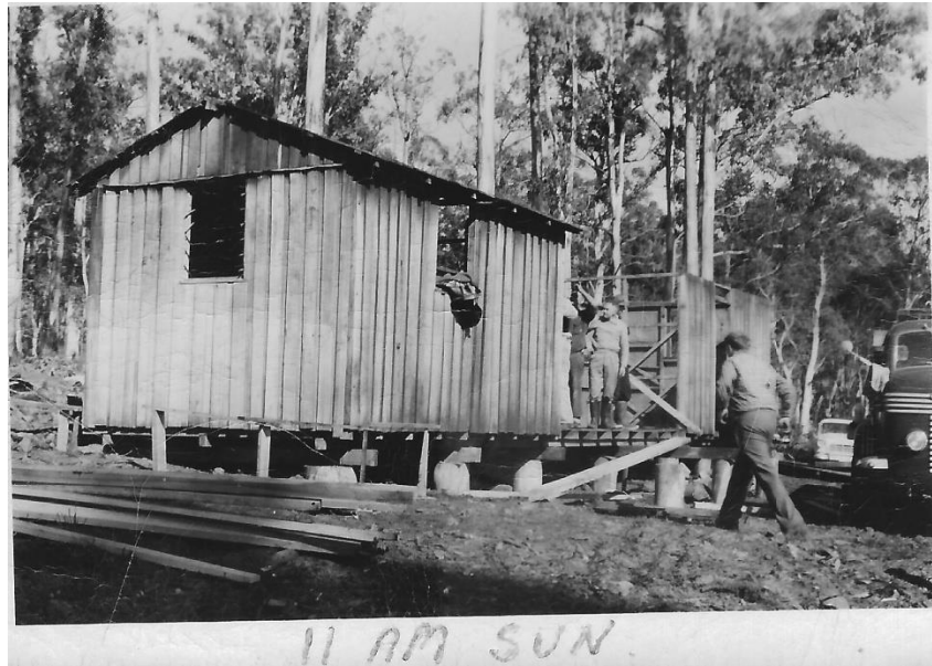
Progress of shack re-erection showing foundation stumps and Commer truck to right, Sunday 5 October 1958, 11.00 am
