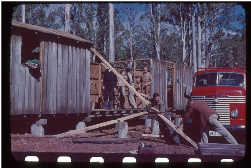
Propping the wall of Dee Lagoon shack during re-erection, Sunday 5 October 1958 (photo: Ray Longden)
