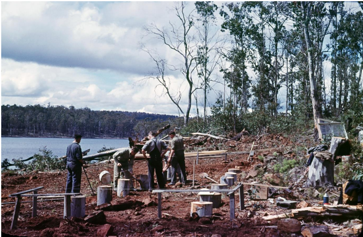
Installation of stumps to receive shack 4 October 1958 (photo: Ray Longden)
