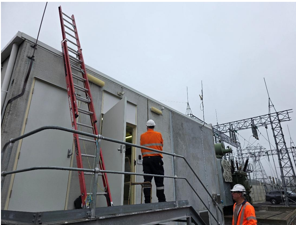
Image: View from South showing existing door and stairs
