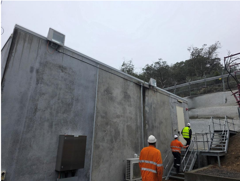
Image: View from North – Showing the higher side of the building
