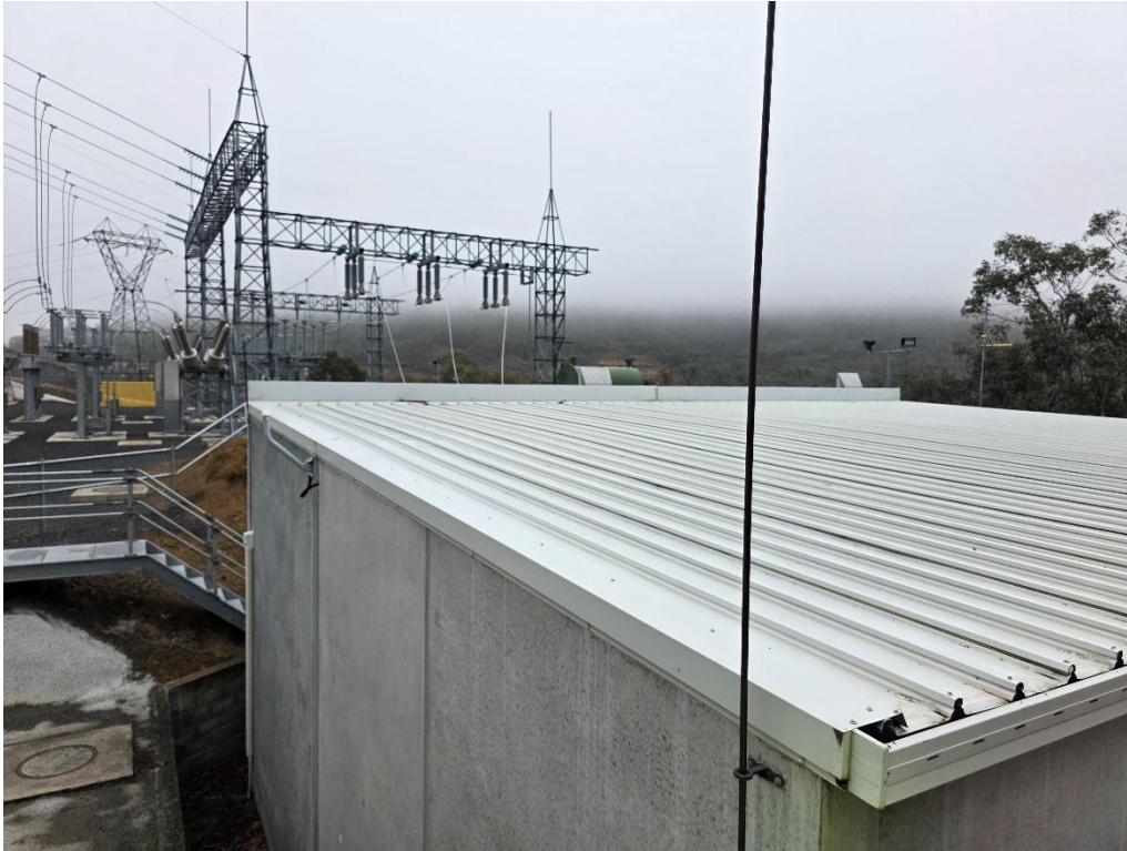
Image: Roof of existing building to be demolished
