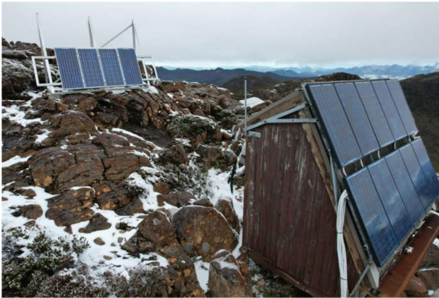
FIGURE 5 INTERNAL VIEW OF SITE SHOWING PARKS AND WILDLIFE (PWS) HUT AND ADDITIONAL SOLAR ARRAY
