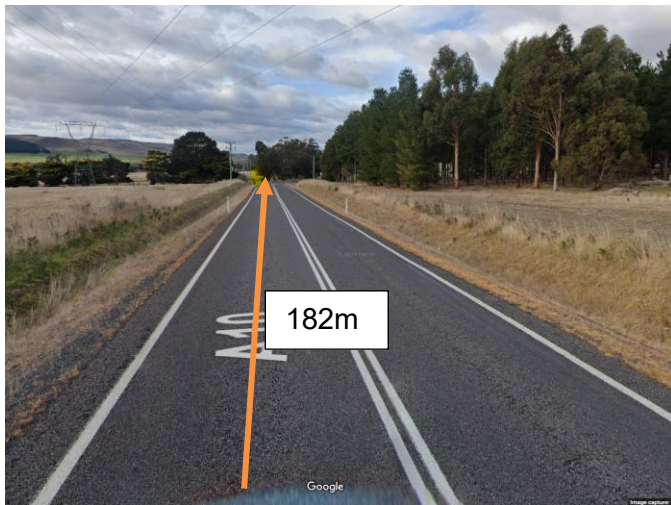
Figure 06: SISD From 182m North to the Intersection
