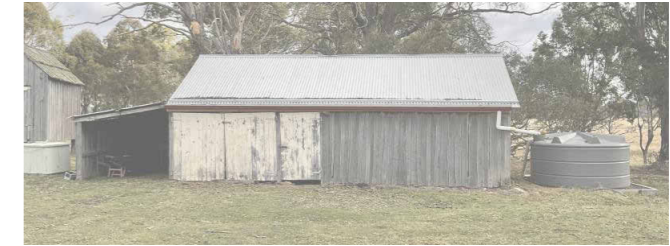
EXISTING OUTBUILDINGS 'A' & 'B' - FROM NORTH
