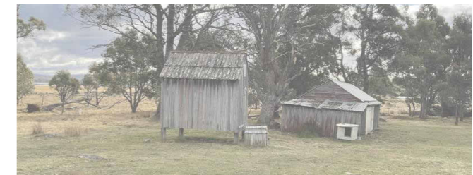
EXISTING OUTBUILDINGS 'A' & 'B' - FROM NORTH
