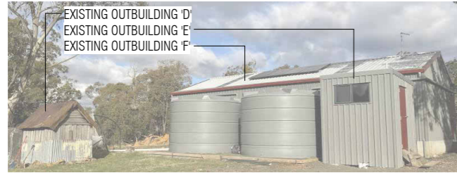
EXISTING OUTBUILDINGS 'D' - 'F' - FROM NORTHWEST
