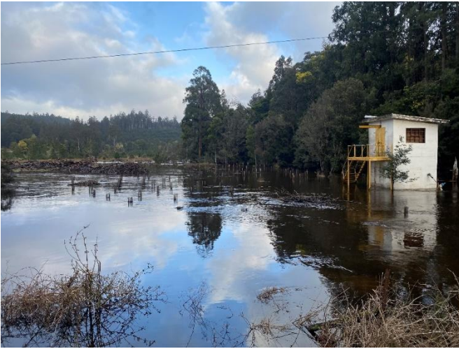
Flooding on the Tyenna River 2024.
