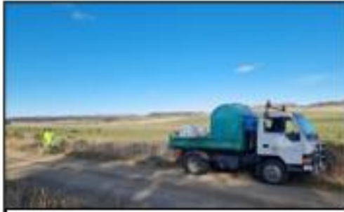
Roadside treatment on Denniston Road
