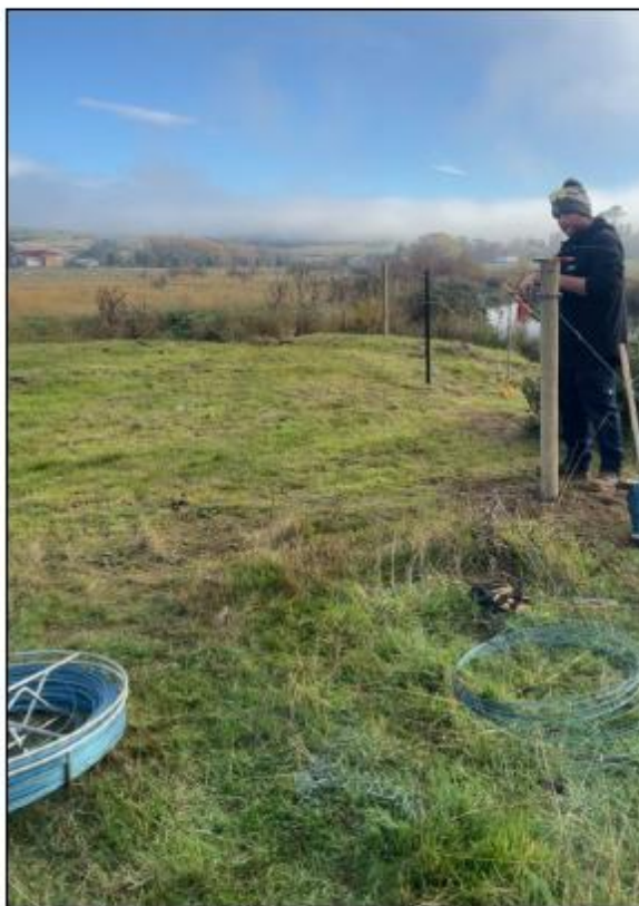
Figure 8. Ouse River restoration project fencing installation
