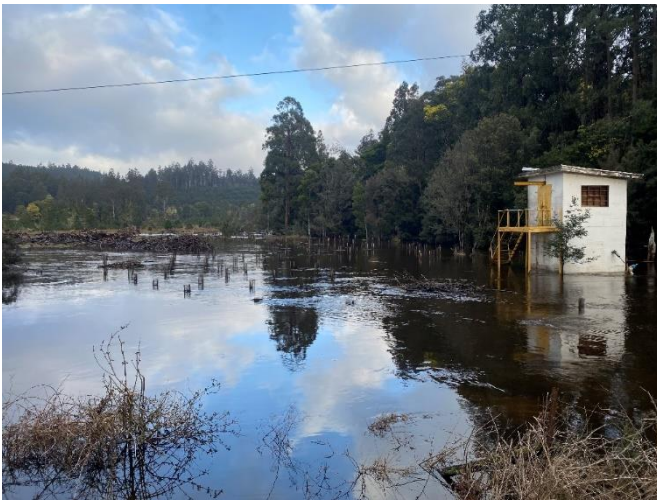
Flooding on the Tyenna River 2024.
