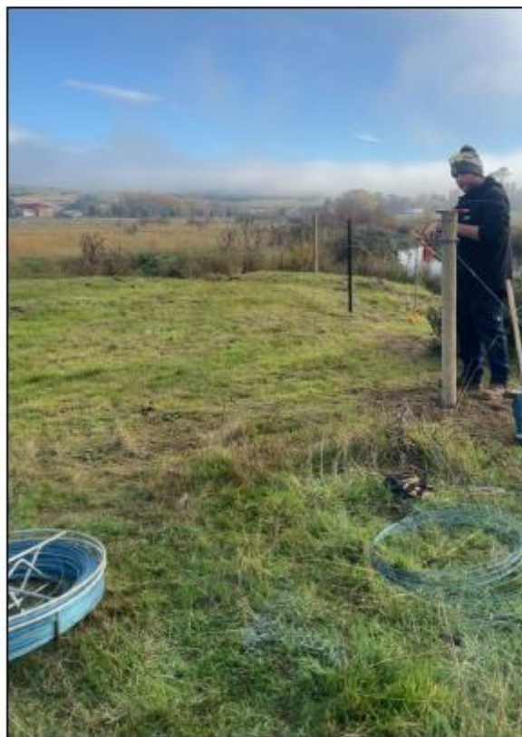
Figure 8. Ouse River restoration project fencing installation
