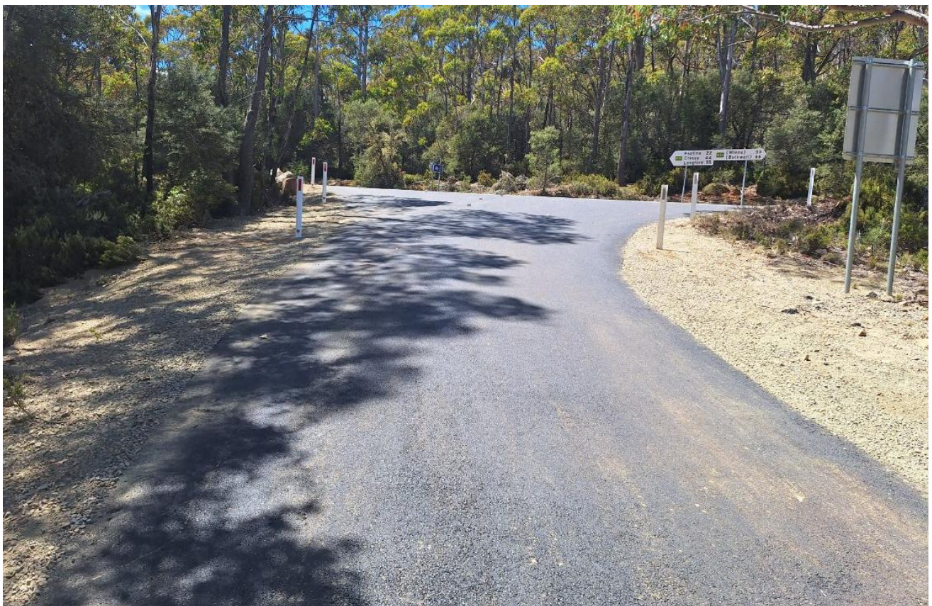
Construction of the junction at Cramps Bay
