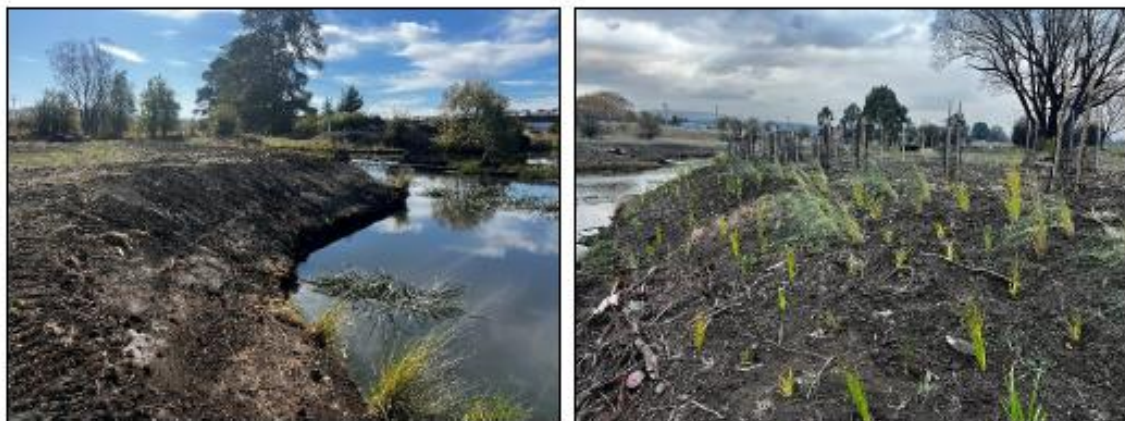
Figure 4. Riverbank stabilisation plantings
