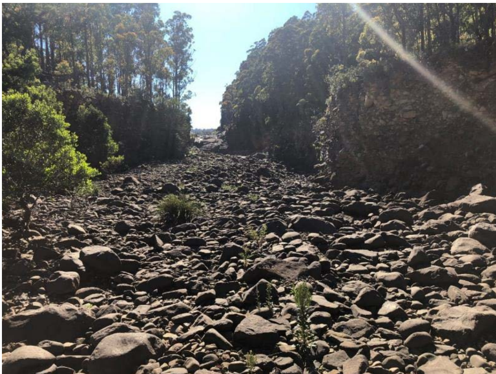
Figure 6.74: Spillway channel connecting Wayatinah Dam to the River Derwent with B. australis plant growing in the middle foreground.
