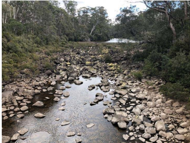
Figure 6.28: Dry riffle immediately downstream Derwent Pumps Weir, isolated pool in foreground. Terrestrial vegetation, mainly woolly tea-tree, has encroached into the channel margins (January 2019)
