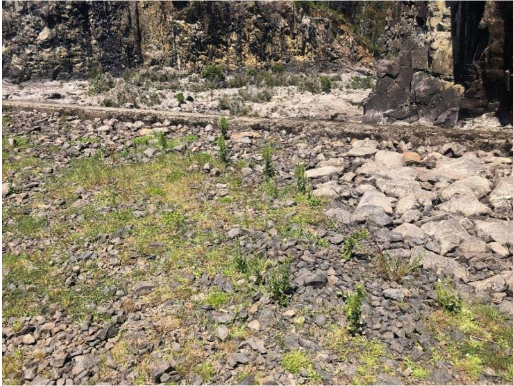
Figure 6.73: B. australis growing along the top of the Wayatinah Spillway.
