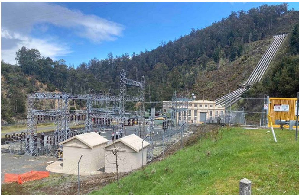
Photograph 2 Historic Tarraleah power station in background with proposed site for new station in the foreground (Source: Inspiring Place)
