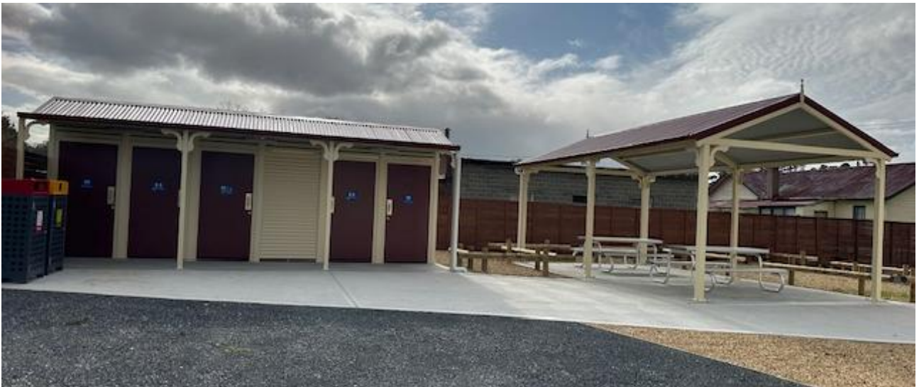
Picture – Ouse Public Toilets
