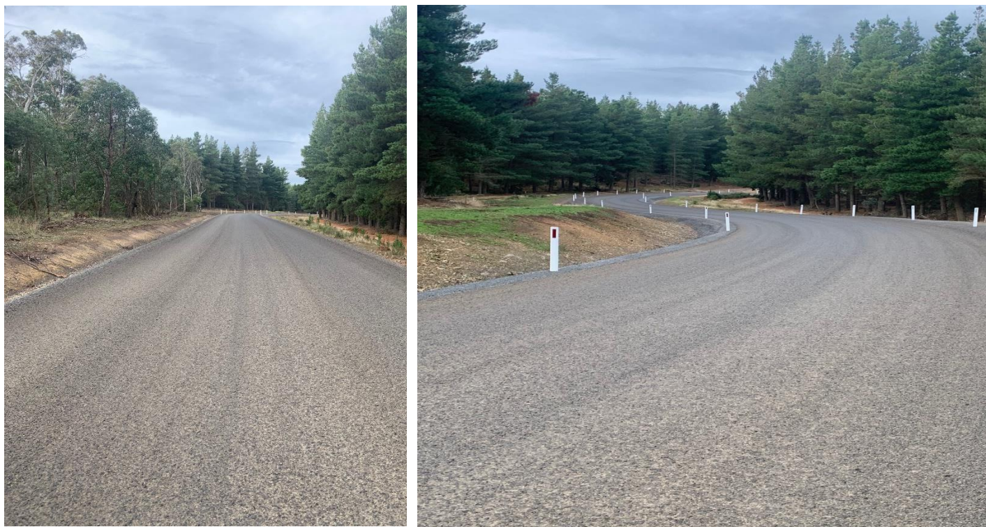
Picture: Road upgrades Stage 4 and Stage 5 on Pelham Road
