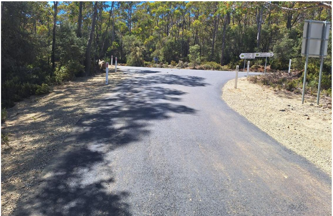
Construction of the junction at Cramps Bay
