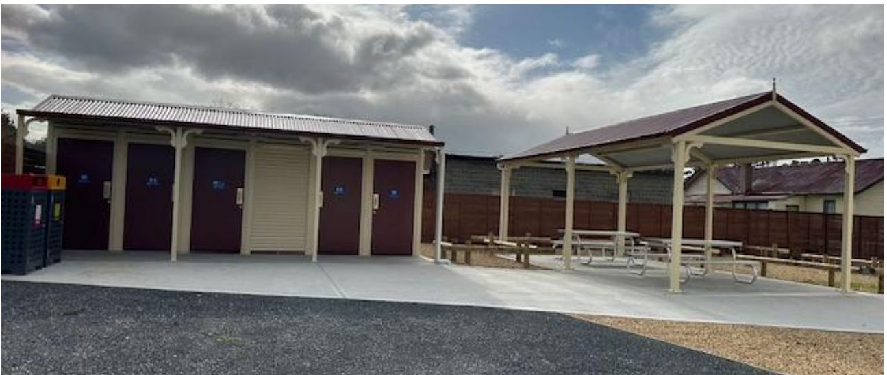
Picture – Ouse Public Toilets
