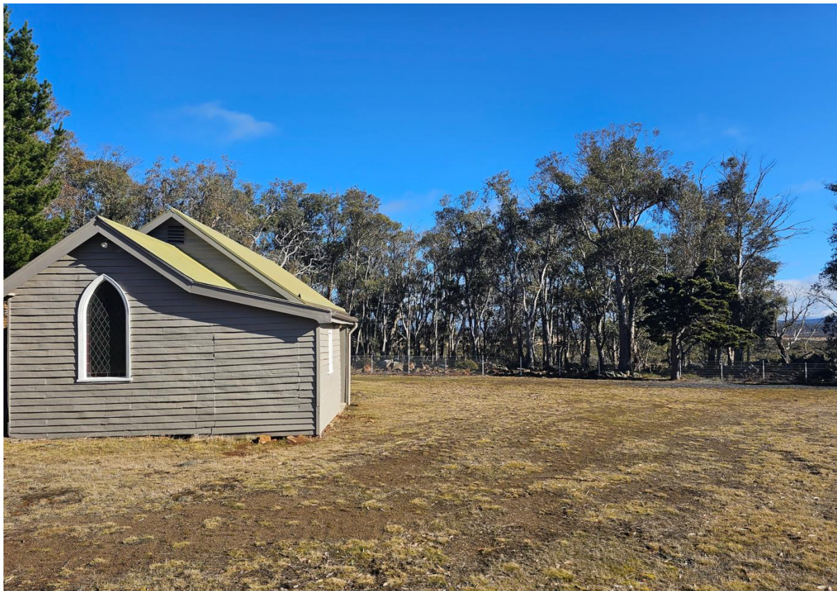
Figure 2.2a - State Heritage Registered (THR No. 10174) Steppes Hall. At this location, WTGs are located to the south or further to the north and not within proximity of the site which means no shadow flicker, according to the submitted Assessment. It is observed that whilst not on the same title, the Hall is surrounded by established Eucalypts and other trees that prevent the site having unimpeded views across St Patricks Plains. (Image: T Henderson, 8 Aug 2023)
