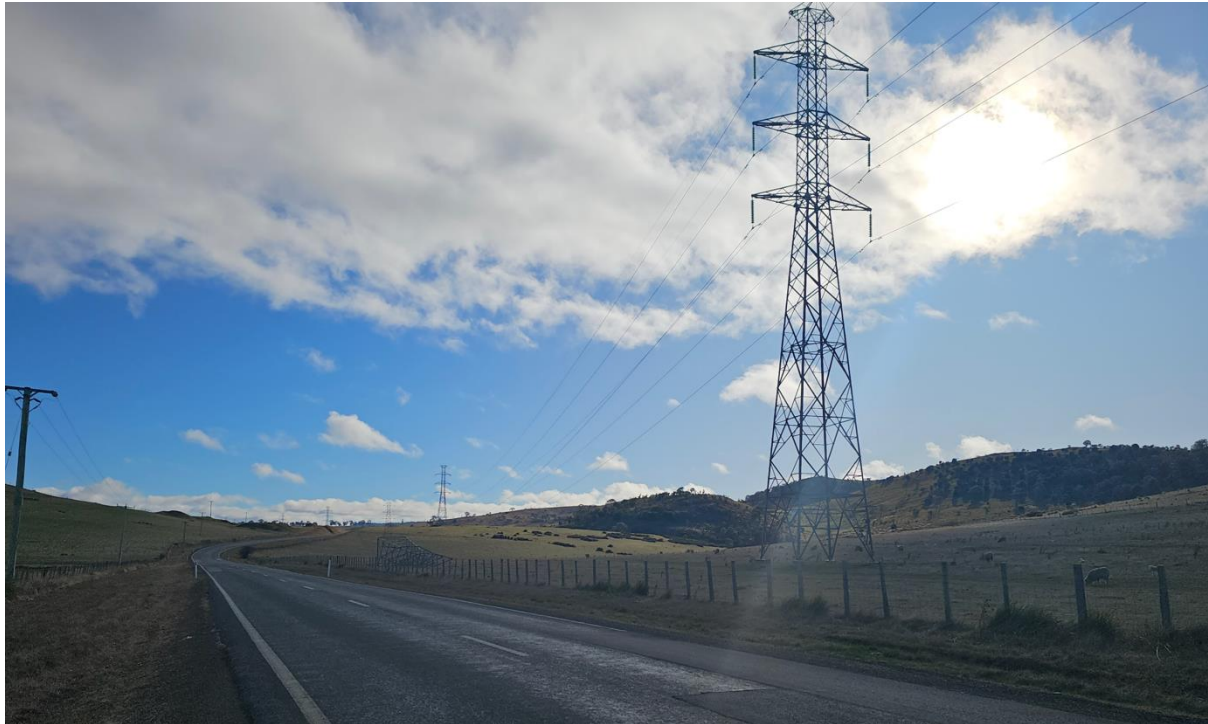
Figure 2.3c - Travelling north along the Highland Lake Road, the high-voltage transmission lines are a feature of the landscape. The structures and associated cables regularly cross the carriageway or run between Bark Hut Creek and just past the southern junction with Waddamana Road. Although not verified, these towers appear to be 50m in height. (Image: T Henderson 8 Aug 2024)
