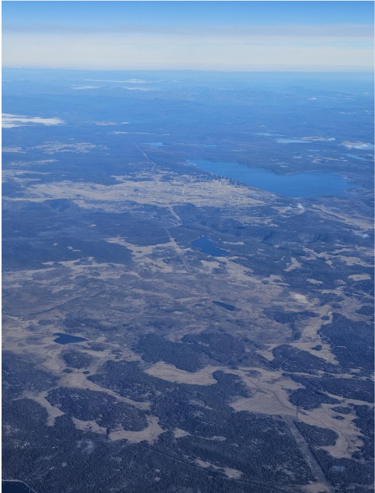
Figure 1.1a – Looking south over St Patricks Plains in the foreground towards the established Cattle Hill Wind Farm in the centre of the image next to Lake Eco. The Shannon River is seen crossing the image with the straight easement for the Transmission Line to Launceston evident. (image: T Henderson 12:56pm Sunday 26 May 2024, aerial view looking south).
