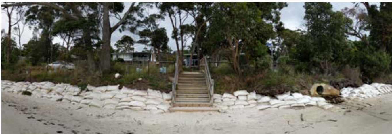
Sandbags provide interim protection for 65 metres of coastline at Coningham Beach in Kingborough Council.
