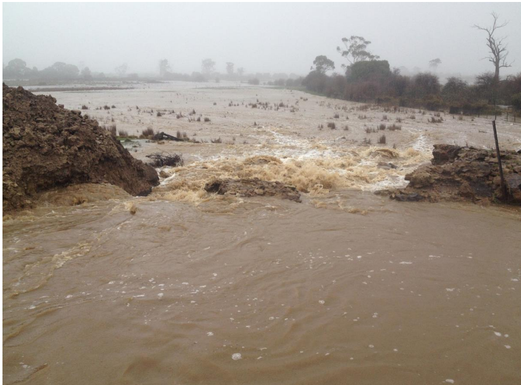
Photo - Flood damaged dam fill infrastructure and inundated farm land, off Lower Farm Road
