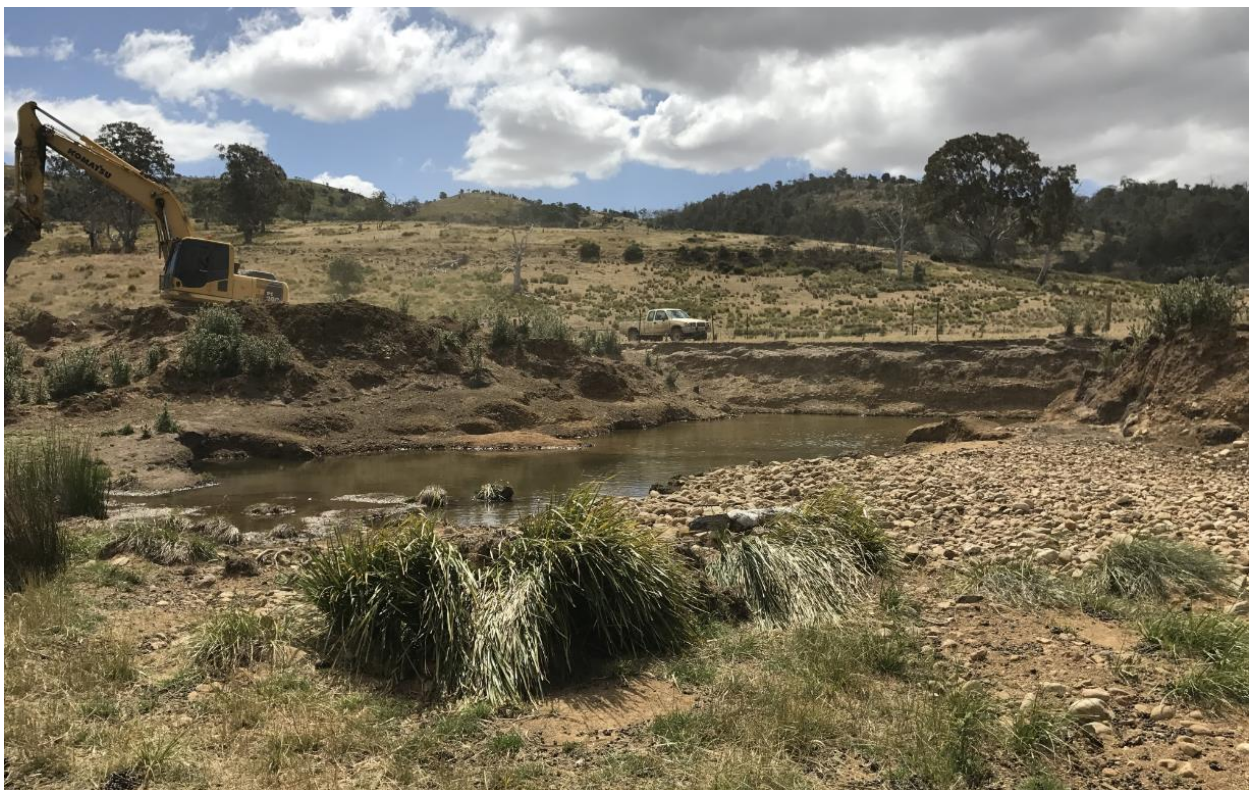
Photo - Dam fill channel completely lost during the 2016 flood event
