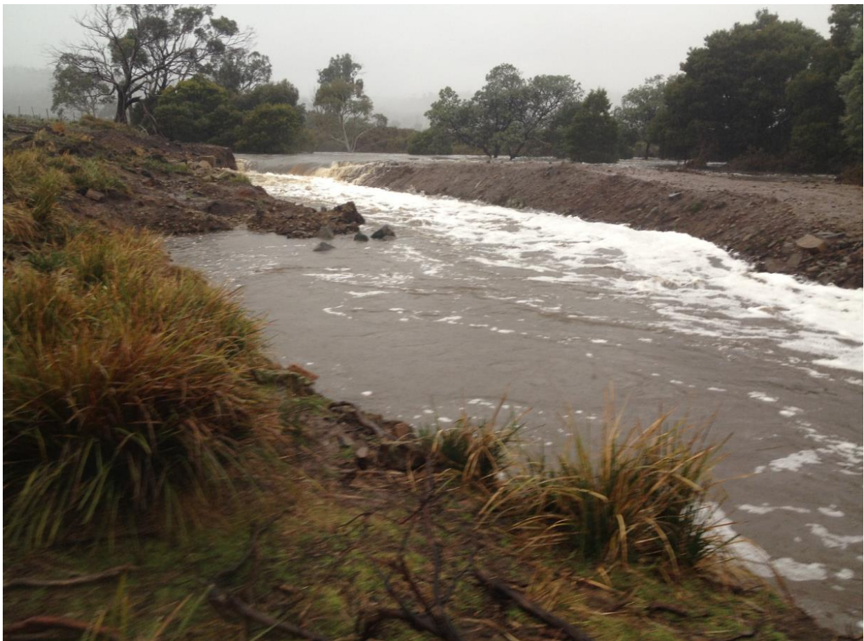
Photo – Clyde River breaching Blair Marsh Dam fill channel, 2016. This breach caused an estimated $200,000 loss in damage to soil and infrastructure on the downstream properties of Lower Farm and Blair. Nine kilometres of fencing was also damaged or destroyed plus three kilometres of deer fencing which had been in place since 1978.
