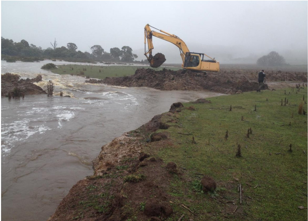
Photo - Excavator being used to divert flood flows to save downstream dams, the wall on the Blair Marsh Dam is 2.4 Kms long and the dam holds 1200 MGL. There was a risk of breaching without the works being carried out with the potential for serious downstream consequences.
