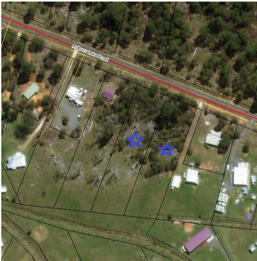
Fig 2. Aerial photo of the subject land and surrounding area, subject land marked with blue stars. (Source: LISTmap)
