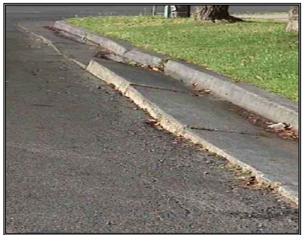
Condition 9 Extreme movement and lack of function
