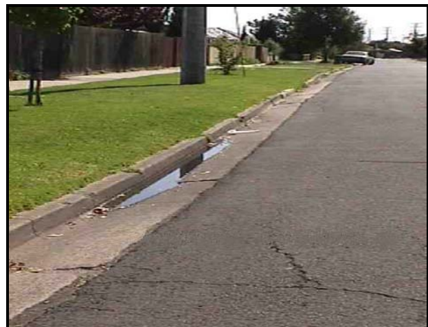
Condition 8 Large movement and holding of water
