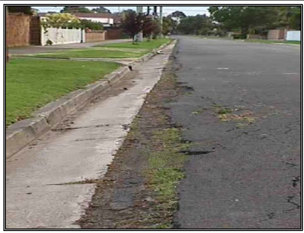
Condition 6 Movement and concrete breakdown
