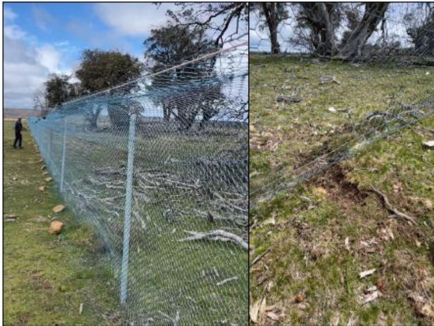
Figure 1. Inspections of the new fence revealed wombat access points, where two-way wombat gates are now being installed.
