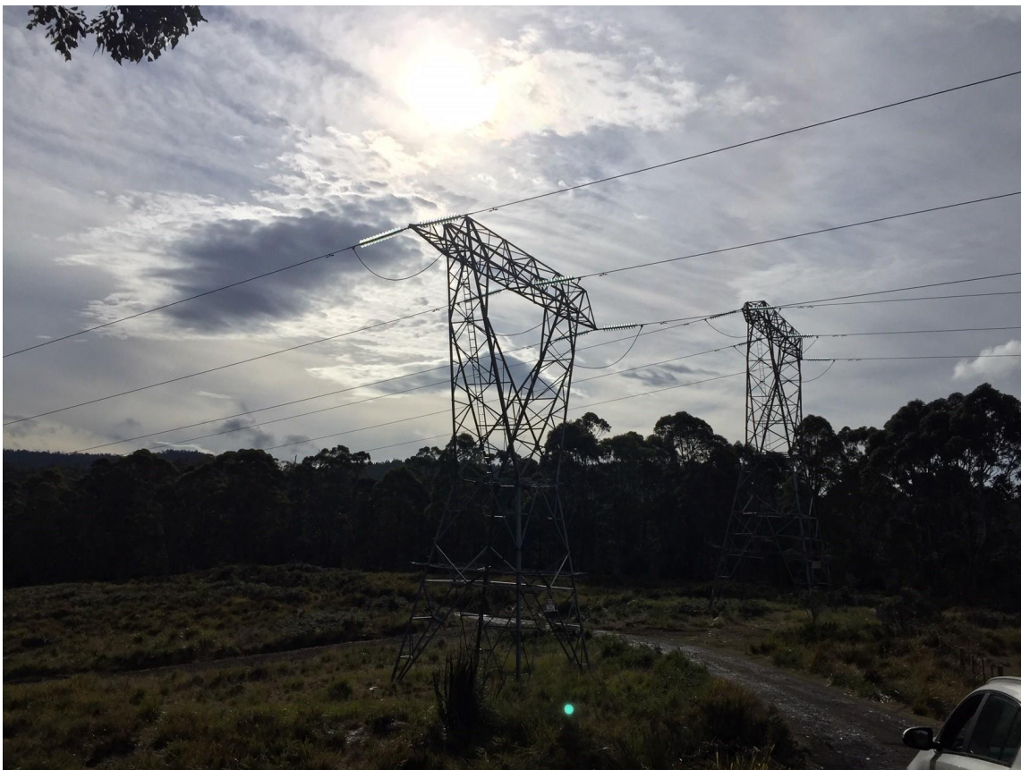
8735 Lyell Highway, Ouse View of the access road on site site, view looking across property to the northern site boundary
