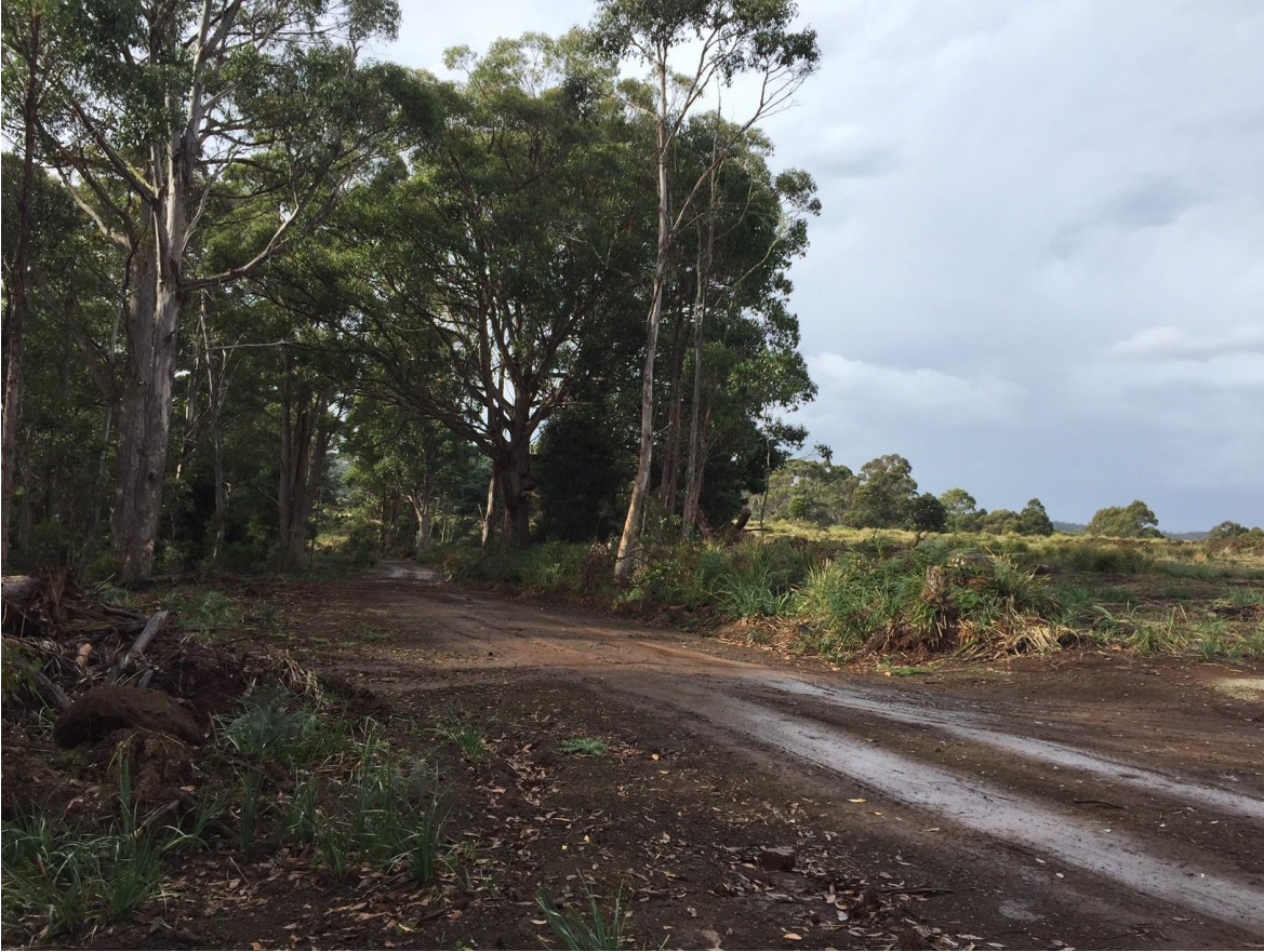
8735 Lyell Highway, Ouse View of the access road on site site, view looking across property to the northern site boundary
