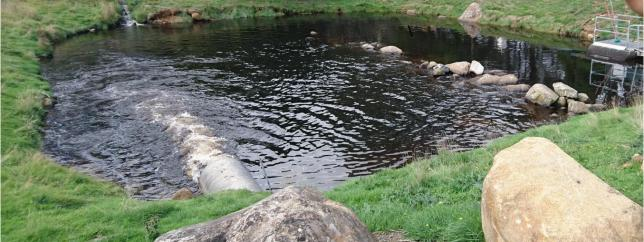
Figure 7. The settlement pond for the Wayatinah Hatchery effluent
