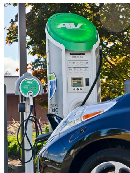
Photo 13. One of many side by side DCFC and Level 2 EVSE installed along the West Coast Electric Highway in Oregon and Washington. Photo from Washington State Department of Transportation (WSDOT).
