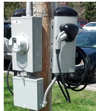
Photo 20. An electrical meter mounted alongside the EVSE and connected with conduit. Photo from NYSERDA.
