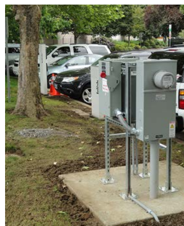
Photo 9. Electrical meter and switch servicing Level 2 EVSE. Photo from Don Karner.
