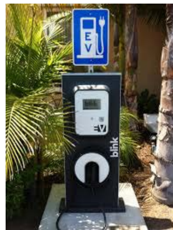
Photo 15. The connector on this EVSE unit is low to the ground to meet ADA accessibility requirements. Photo from Ecotality.
