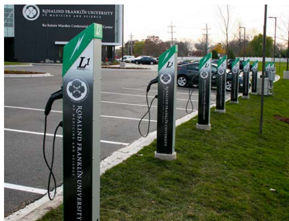
Photo 12. Level 1 pedestal EVSE at Rosalind Franklin University in Illinois. Photo from Telefonix.
