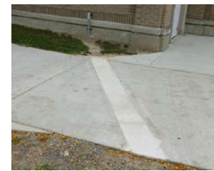
Photo 8. Trenching through soil and sidewalk was needed to install EVSE at the University of Buffalo. Photo from NYSERDA.
