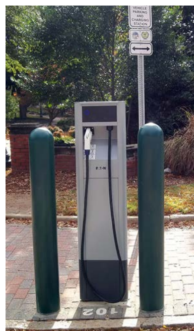
Photo 2. Pedestal-mounted EVSE installed by the City of Raleigh, N.C., for free public use. Photo from Kathy Boyer, NREL 18520
