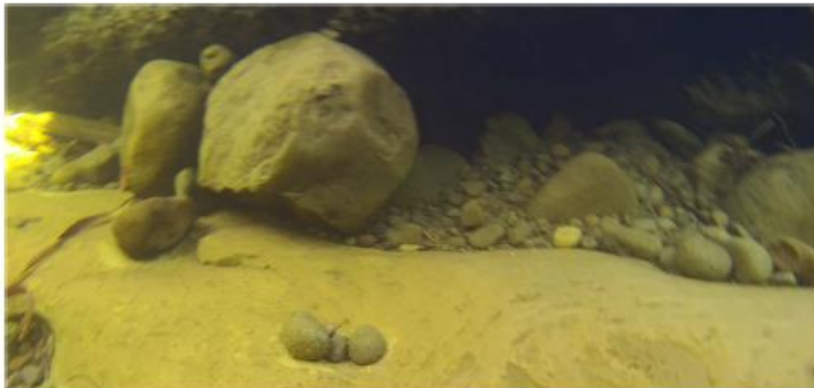
Picture 05 – Further undermining on North Western end of Pier 1
