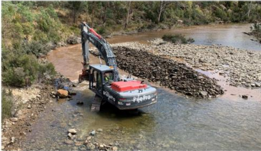
Picture 02 – Further temporary river channelling
