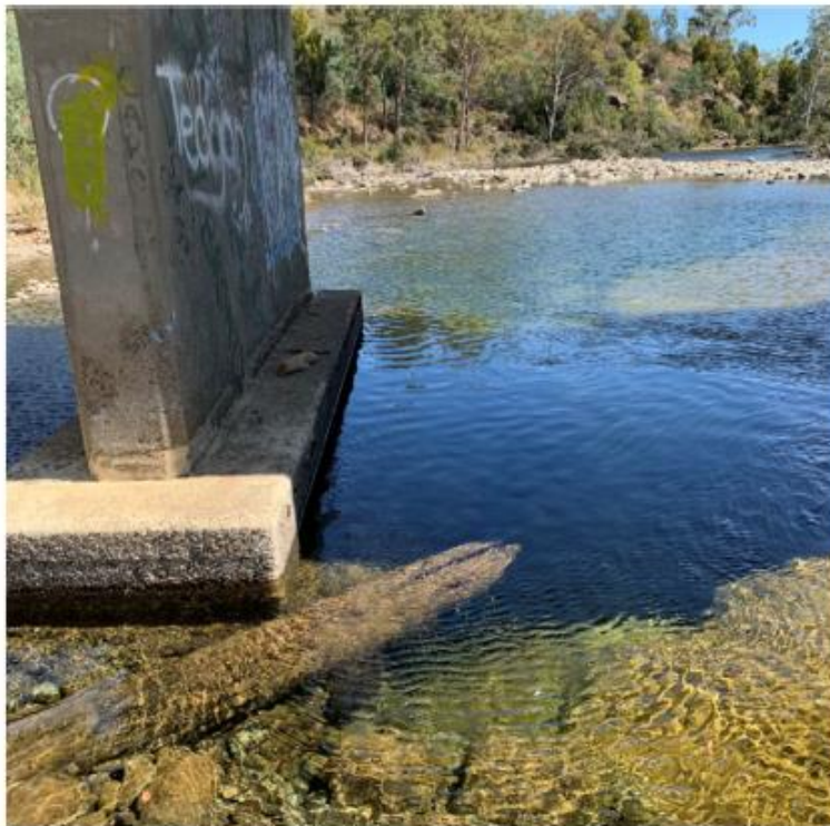
Picture 07 – Another view of the existing undermining
