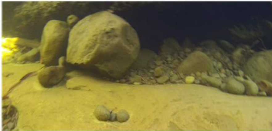
Picture 06 – More Undermining on Pier 1
