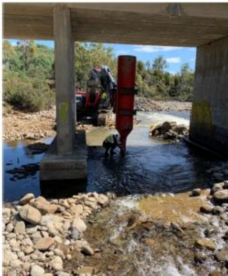
Picture o9 – Kibble Attachment installing concrete
