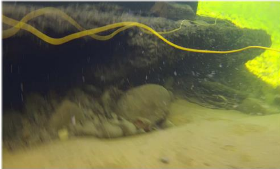
Picture 04 – Undermining on Northern End of Pier 1
