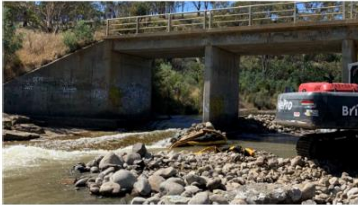
Picture o8 – Silt boom to capture concrete fines
